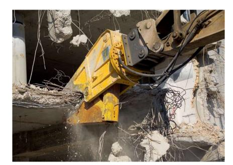
360° endless **hydraulic rotation** allows optimal positioning and precise handing.
