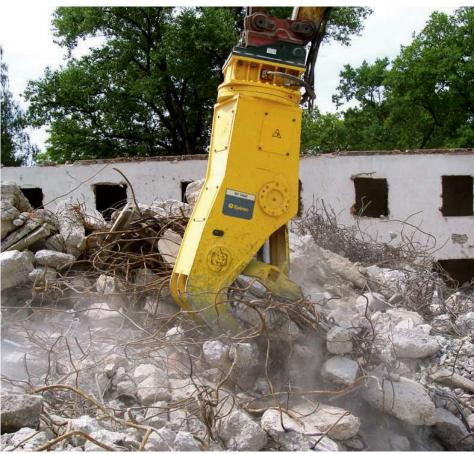
The Bulk Pulverizers' smart design also makes them ideal for primary demolition of ceilings and walls.
